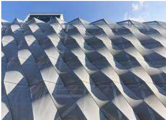
Figure 2: High performing fabric facade
